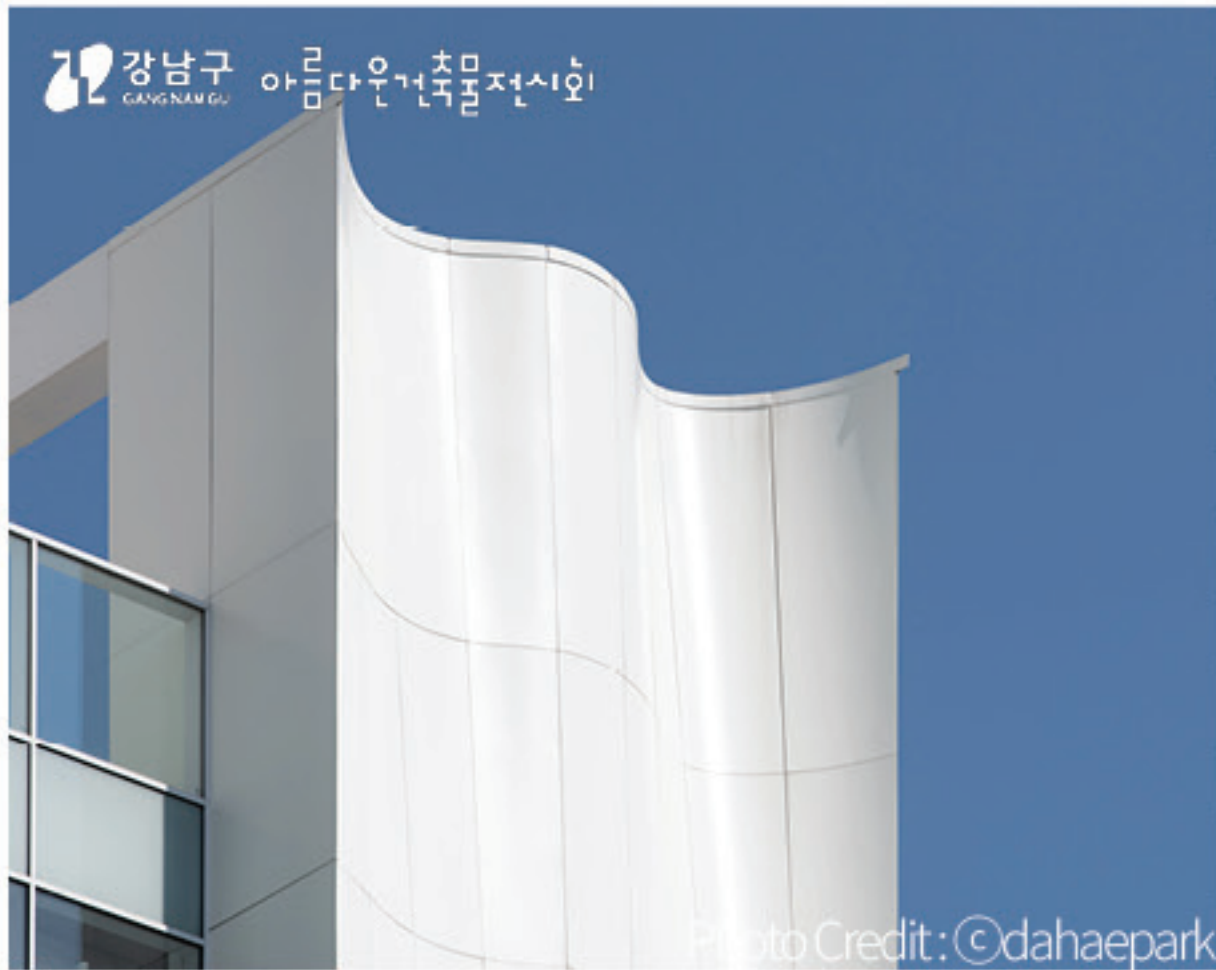
2025 Ripple Tower Nonhyeon-dong, Gangnam-gu, Seoul Built Work
