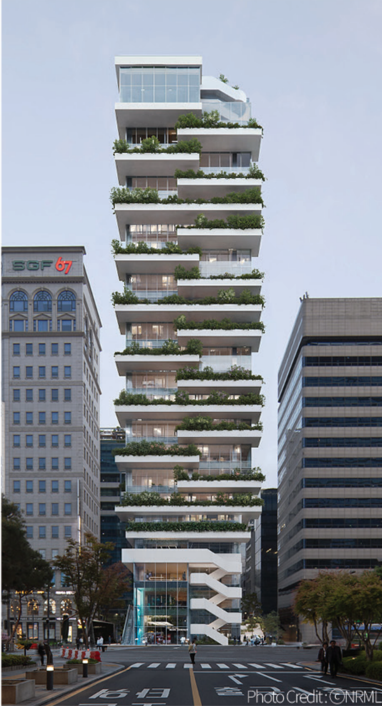
2023 Ripple Tower Nonhyeon-dong, Gangnam-gu, Seoul Under Construction
