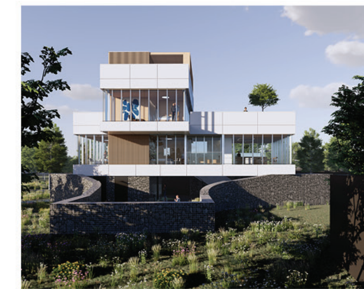
2023 Floating Cross House Hwayang-Myeon, Yeosu Under Construction
