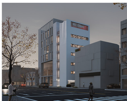
2023 Ripple Tower Nonhyeon-dong, Gangnam-gu, Seoul Under Construction
